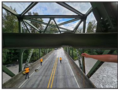
WSDOT has begun installing temporary steel braces to stabilize the SR 410 White River Bridge between Buckley and Enumclaw. These braces will enable crews to make permanent repairs, which is expected to begin the week of Sept. 15, 2025. The bridge will remain fully closed to all traffic throughout the temporary and permanent repair process in order for contractor crews to work safer and more efficiently.
